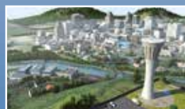
Drinking-water distribution systems
